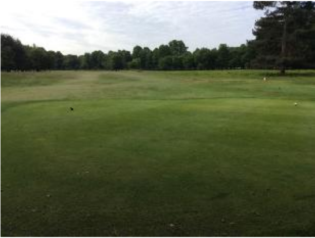
Figure 7: The newly constructed 6 th Tee is an excellent addition providing ample teeing area and superb surface levels. All works were carried out in-house.
